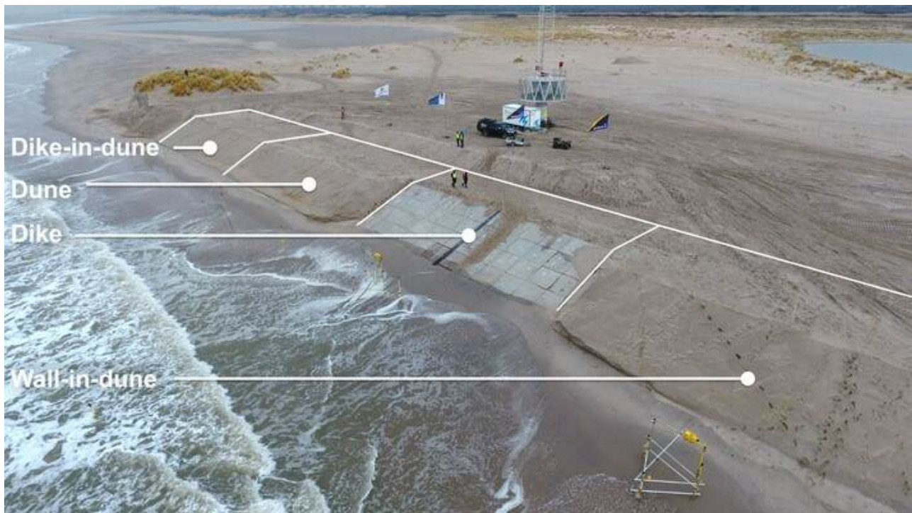
The test setup at the Sand Motor. Just after construction, with the concrete tiles of the dike section visible and the hard elements of the dike-in-dune and wall-in-dune still hidden under the sand.
